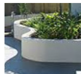
Rendered Masonry
